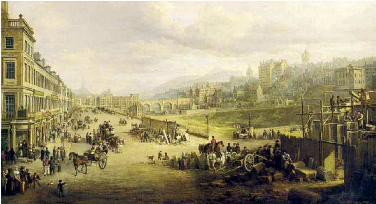
Alexander Nasmyth: Edinburgh from Princes Street with the Royal Institution under Construction , 1825 (cropped to fit).
